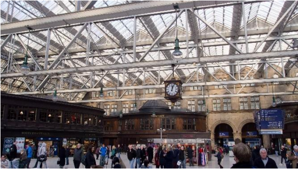
Main concourse truss (“ Glasgow Central railway station ” by Ed Webster, licenced under CC BY 2.0 )
