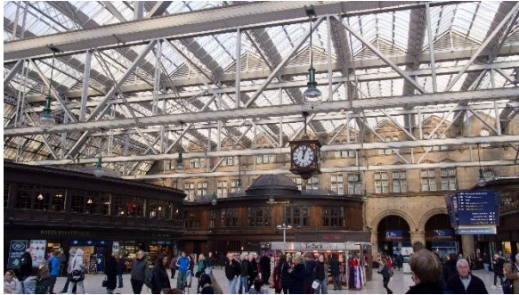
Main concourse truss (“ Glasgow Central railway station ” by Ed Webster, licenced under CC BY 2.0 )
