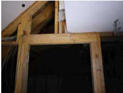
Door lintel beam supporting a roof beam
