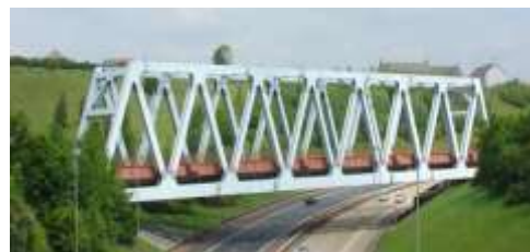
(c) A modern bridge truss
