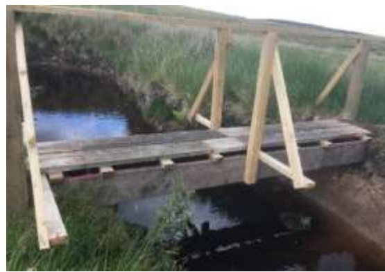
Side view of the bridge
