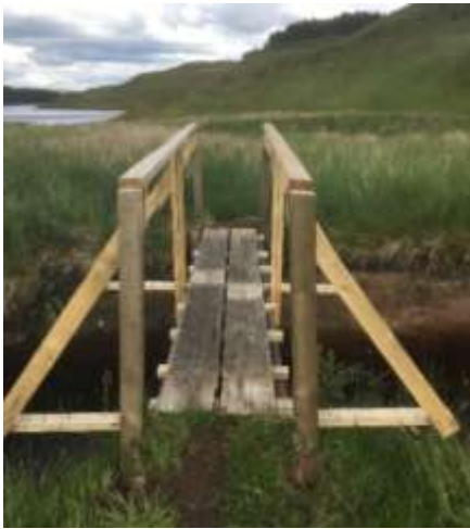
Front view of the bridge
