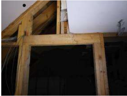
Door lintel beam supporting a roof beam
